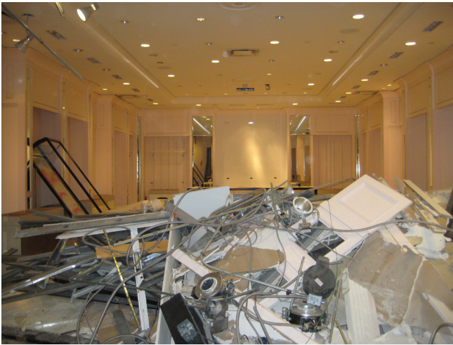
Figure 1. Typical demolition of a commercial interior. Photo by Yarden Harari.
